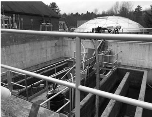
*Newly raised walls are seen on the chlorine contact chamber, which was done to prevent overflow.*
