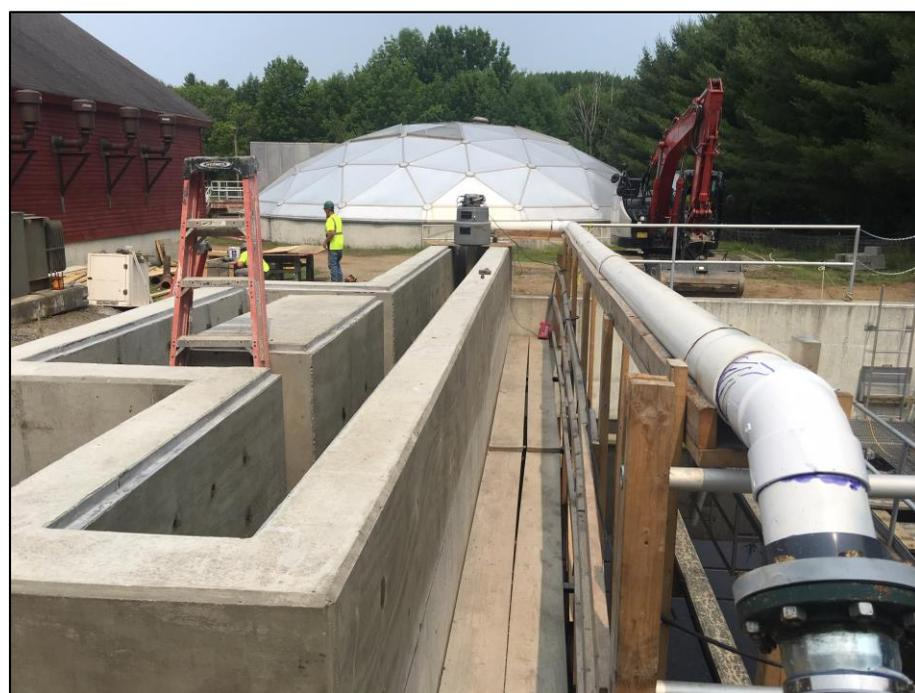
WASTEWATER FACILITY UPGRADES • Temporary bypass piping is seen over the chlorine contact chamber outside the Wastewater Facility recently. The chamber walls are being raised as a preventative measure against overflow and bypass channels are being installed to help streamline maintenance.
